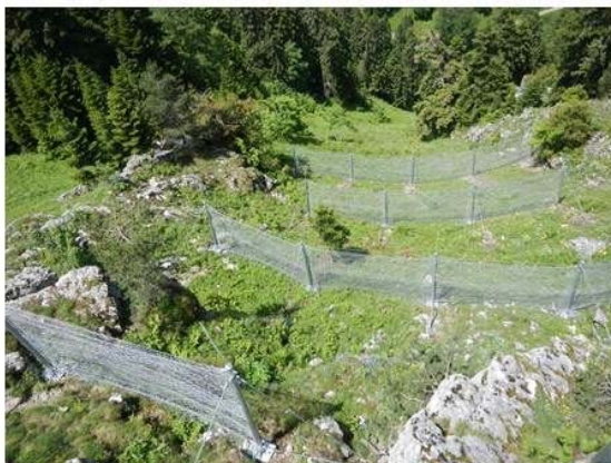
Avalanche Prevention fence installed in Bolu Turkey
