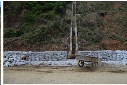
Making the gabion box in October
