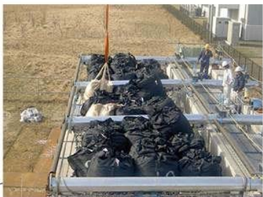
Load test for Sediment soil pressure
