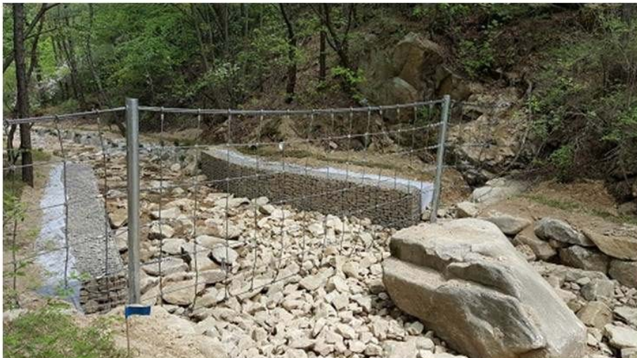
Debris flow barrier installed in Seoul city
