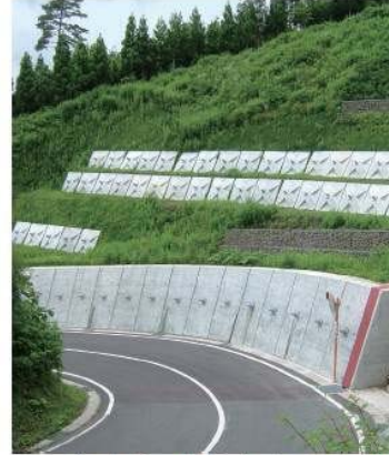
Construction works for forest road restoration
