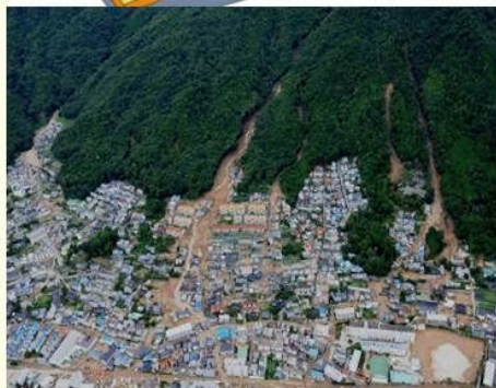
2014.8 Hiroshima Landslide Disaster
