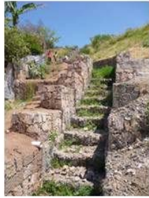
Drainage with gabions
