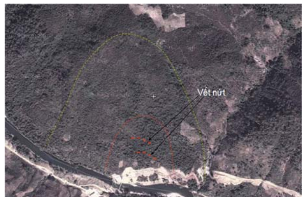
Figure 6: Landslide at Nam Non Bridge, West Nghe An road, My Ly commune, Ky Son district, Nghe An province
