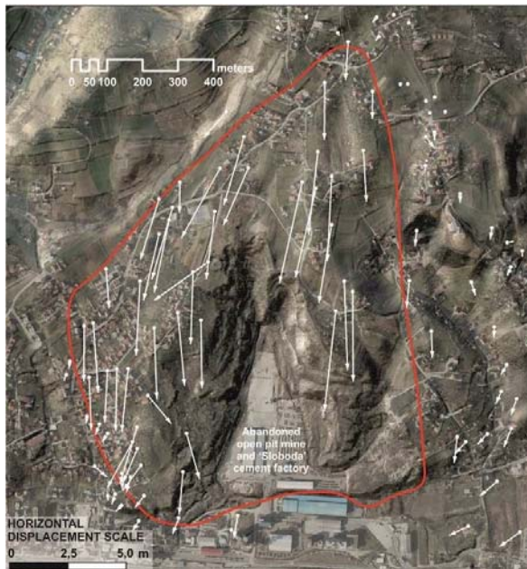
Figure 8 Horizontal displacements (white arrows) at the Kostanjek landslide area in the period 1963-1988 based on interpretation of stereo pairs of aerial photographs from 1963, 1979, 1981, 1985 and 1988 (Ortolan and Pleško 1992). Red line depicts the outline of the Kostanjek landslide according to interpretation by Ortolan (1996). In the background is orthophoto image from March 2012. Devastated slopes of the abandoned open pit mine are clearly expressed by rough relief forms in the middle of the Kostanjek landslide. The former cement factory 'Sloboda' was placed in the plain area in the bottom middle part of the landslide.
