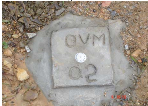
Figure 12 Concrete post for landslide monitoring
