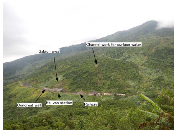
Photo 1 Topology of Hai van station landslide area
