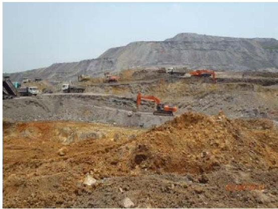
Fig. 5 Dump site area after the landslide
