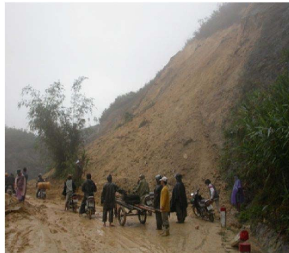
Figure. 7 Landslide at section 1
