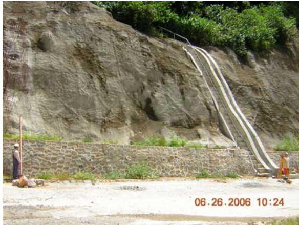
Figure 13 Geodetic measurement for landslide movement
