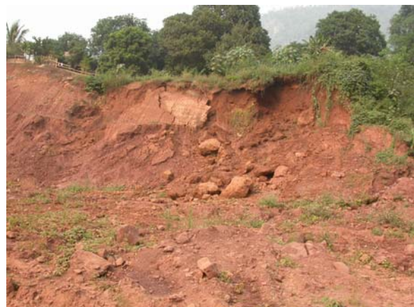
Figure 7 The topple in national road No.6
