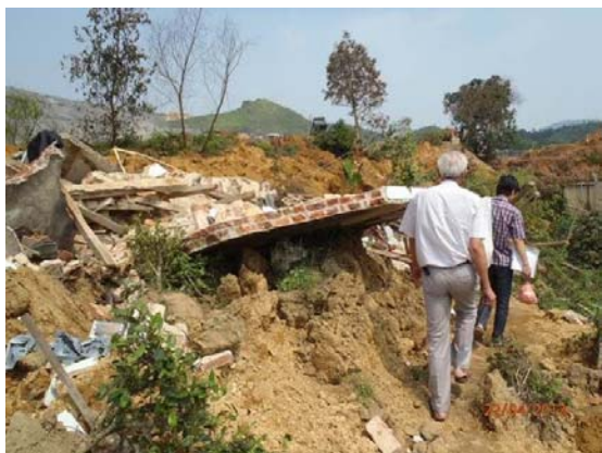
Fig. 6 A house was completely destroyed
