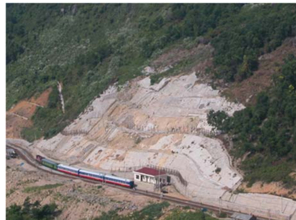
Figure 9: Location landslides at Hai Van Pass station
