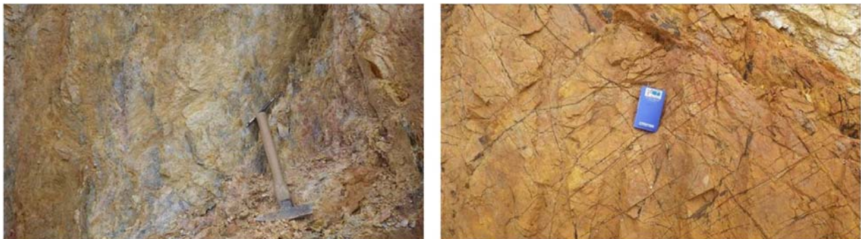
Figure 16 Cracks (right) and faults (left) at No. 485
