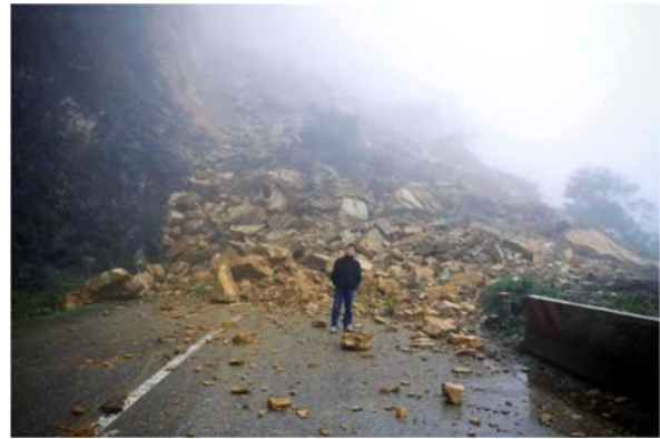
Figure 5: The rapid slope failure at Km 138 +750, Dong Bang Commune, Mai Chau District, Hoa Binh Province
