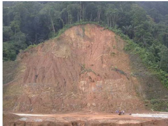
Figure. 10 Landslide at section 4
