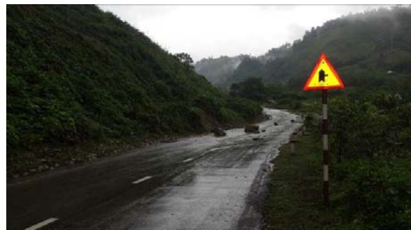
Figure 29 Rock fall in the hornfels distribution area (No.20)
