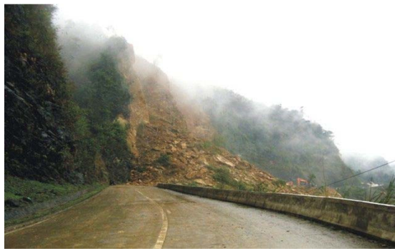
Figure 5 Landslide on Highway No.6, 2012
