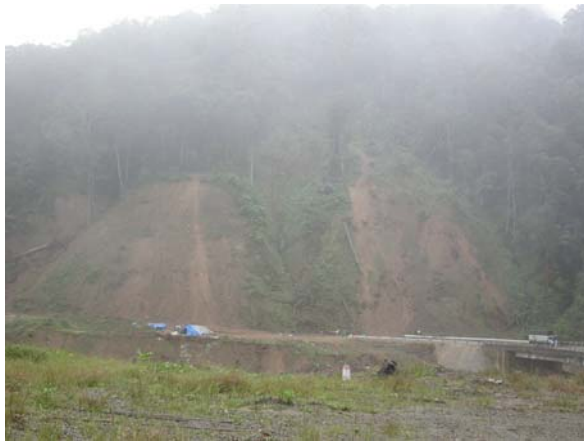
Figure. 8 Landslide at section 2
