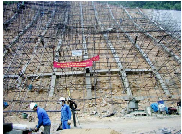
Figure. 11 The landslide prevention by using OVM anchor reinforce
