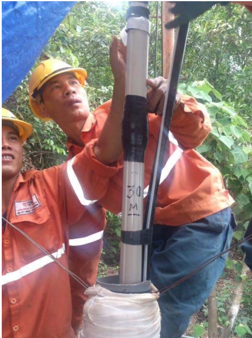
Figure 16: Install inclinometer casing and insert tube to pump grout
