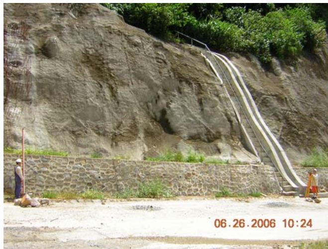
Figure 13 Geodetic measurement for landslide movement
