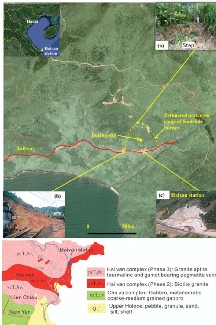
Fig 1. Location, topography, landslide border and geological structure of Hai Van station landslide, Danang city, Vietnam (a: a small step where a head scarp of a landslide may be formed; b: previous landslide in 2007; c: Hai Van station)
