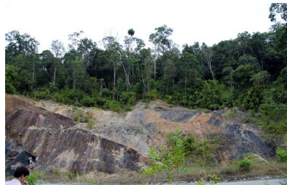
Fig.5.4 Photo of Translational rock slide Northwestward of Thach My town
