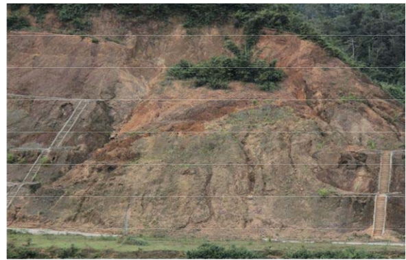
Fig. 5.5-b Photo of main scarp of a rotational landslide in HCMR (Quang Binh section)
