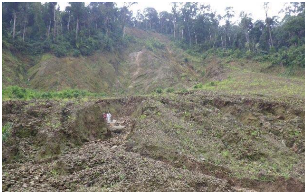
Fig. 5.5-a Photo of landslide body of a rotational landslide in HCMR (Quang Nam section)
