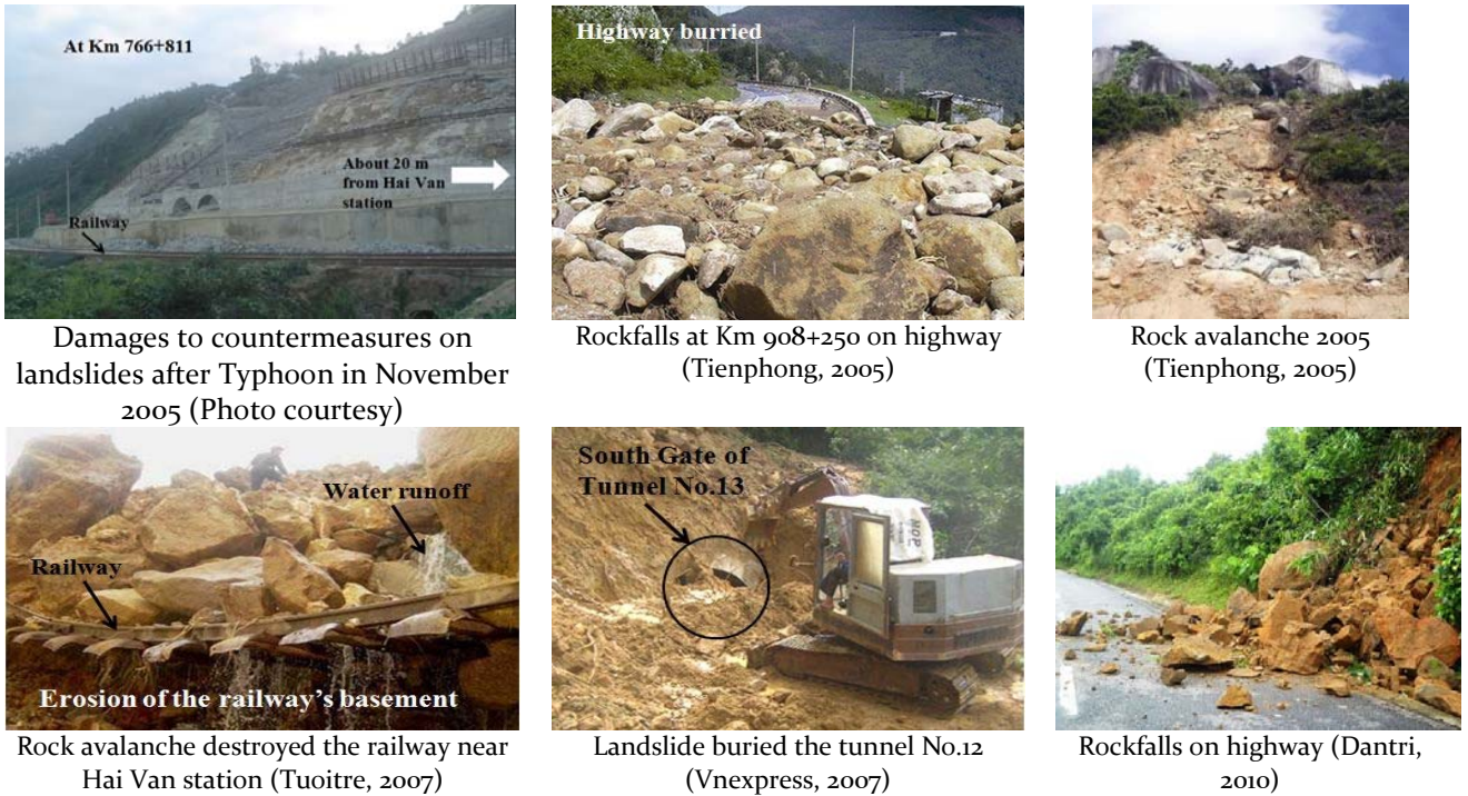
Figure 2 Photos of several landslides and its impacts
