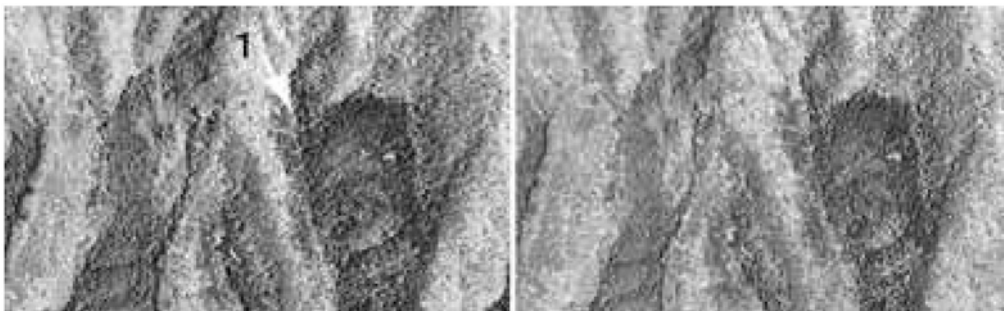
Figure 22 Landslide body and adjacent environment. Landslide body at lower face to the other near. Decreasing (stabilizing order). Weight value: 0.9. The landslide body moved but if it stop by any barrier the potential of reoccurrence should be decrease (Miyagi et al., 2004).
