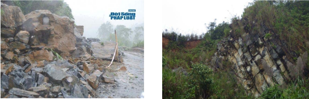
Fig. 5.1 Rockfall on HCMR– Quang Nam section – Vietnam
