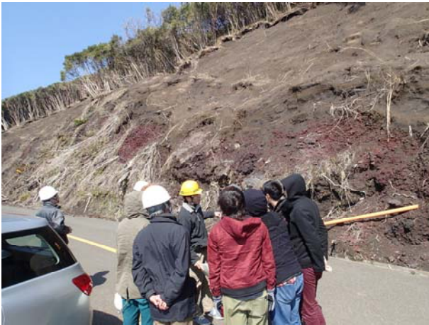
Figure 1 Field investigation in the collapse area
