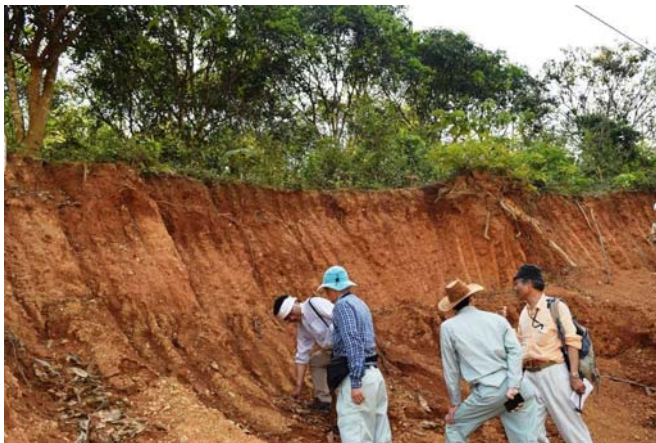
Fig. 1 Landslide field survey along the National Road No. 7 (May, 2016)
