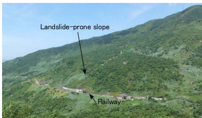
Fig.2 Landslide slope in Hai van Station (Asano et.al.2016)
