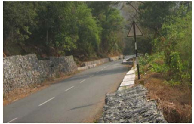
Figure 9 Gabion walls constructed along Mettupalayam – Coonoor highway
