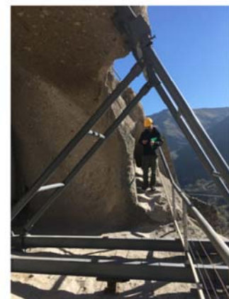
Temporary scaffolding to support unstable block before the final consolidation (anchors and passive bars – spring 2019)
