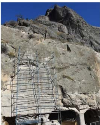
Temporary scaffolding to support unstable block before the final consolidation (anchors and passive bars – spring 2019)
