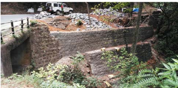
Figure 2 Gravity retaining wall constructed along Mettupalayam - Ooty Highway
