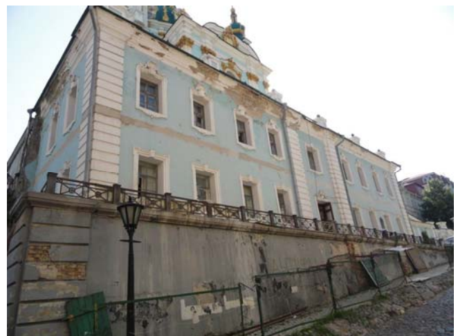
Figure 7 General view of the church superstructure and the runway construction.
