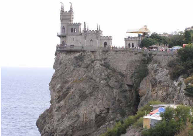
Figure 1 Swallow's Nest castle. South-west view. The crack in the cliff is obvious (the crack width is up to 0,5 ~ 0,7 m).
