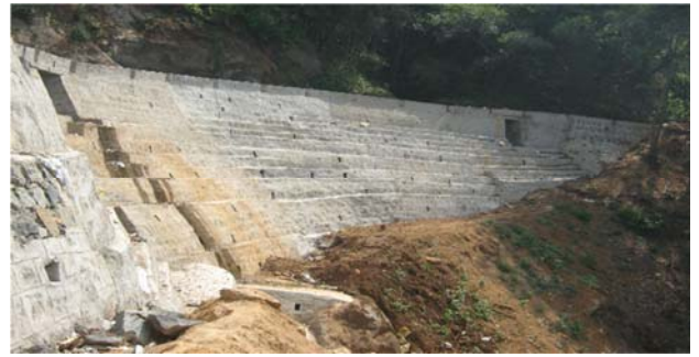
Figure 3 Retaining wall at Marappalam 2009 landslide location
