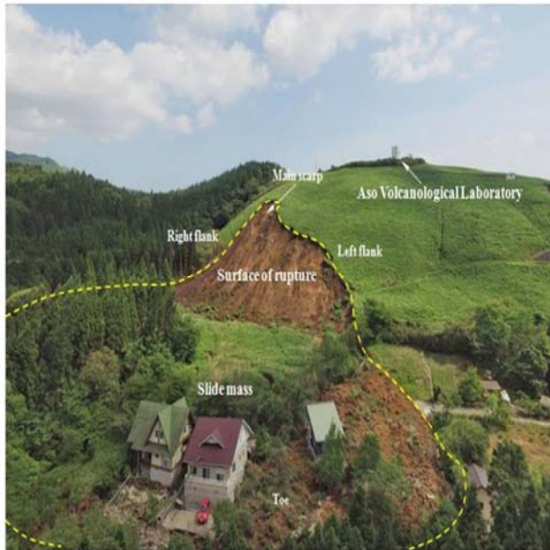
Oblique aerial view from the toe of the landslide towards the source area
