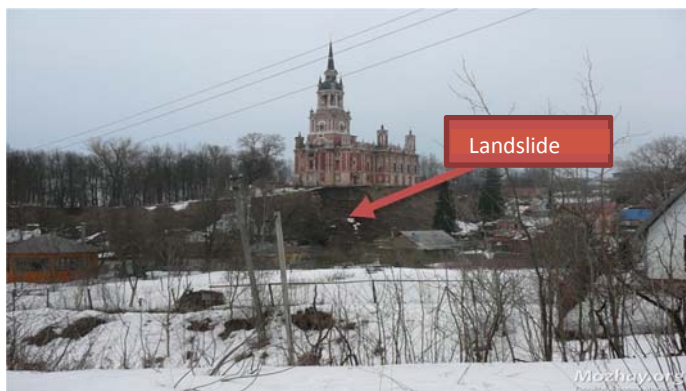
Fig.6 The landslide near the south-western corner of the Novo-Nikolsky Cathedral.
