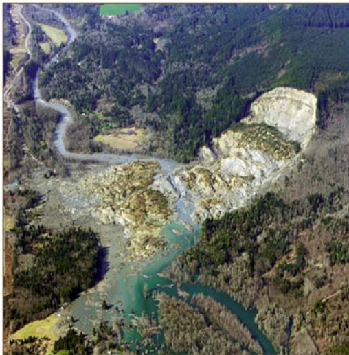
rainfall induced, Oso landslide, Washington, USA
