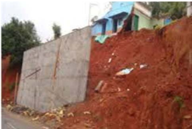
Figure 8 Cantilever retaining wall at Ooty
