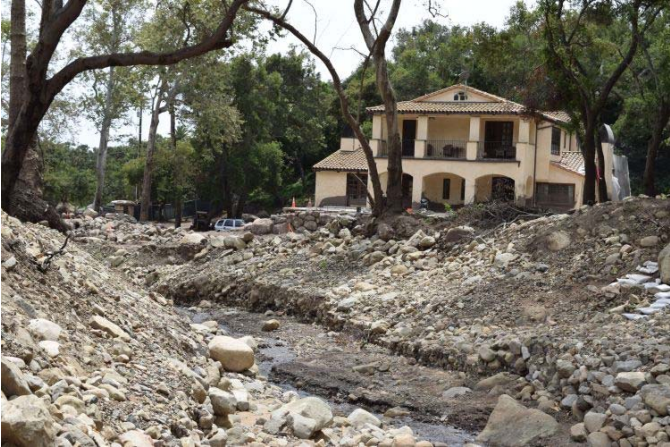
Figure 2 Damage to buildings due to the debris flow and damage of culverts/bridges.
