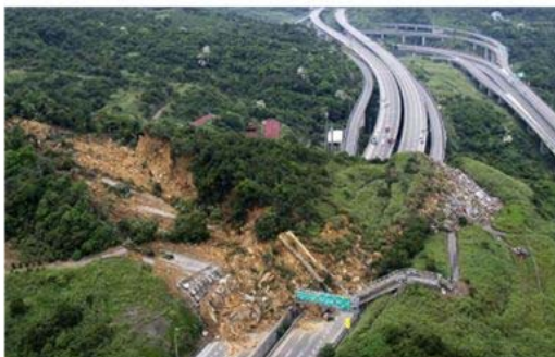
Hazards to Transportation
