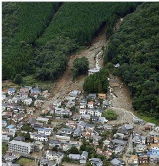
Hazards to Residents
