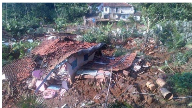
Figure 1 Landslides due to high rainfall in Banjarnegara , Central Java
