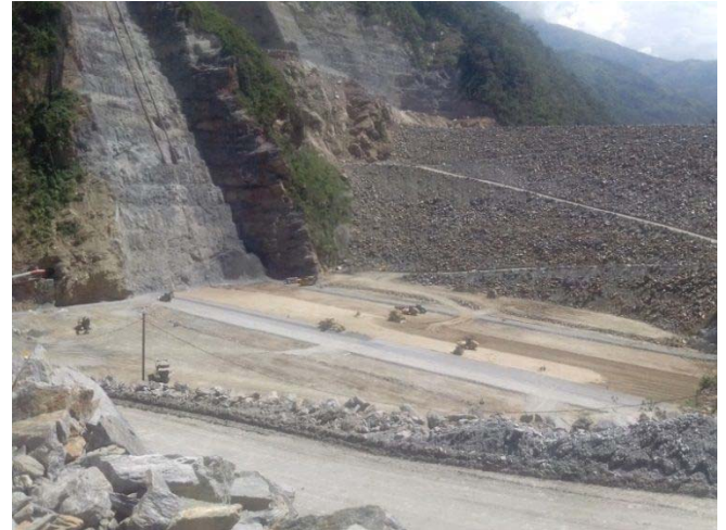
Figure 4. Photo of the dam construction process (Cortesy of R. Moreno).
