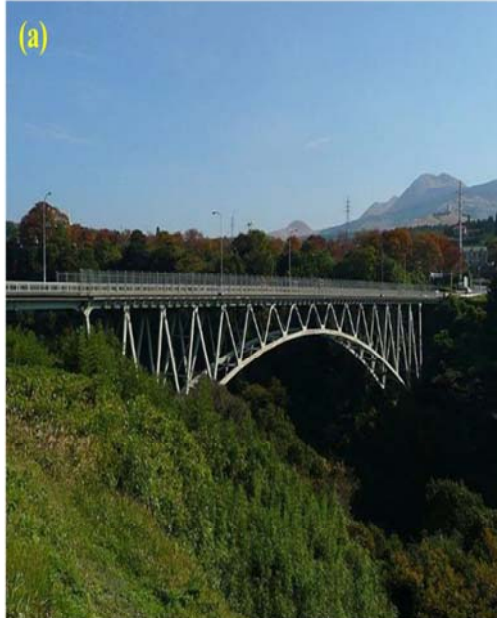
Aso bridge before landslide
